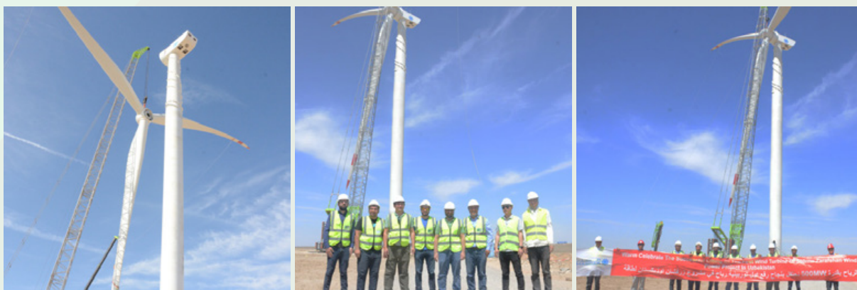
Installing the first wind turbine of the 500MW Zarafshan Wind Power Project
