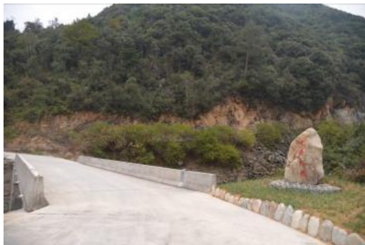
Picture: "BOC Bridge" was completed
