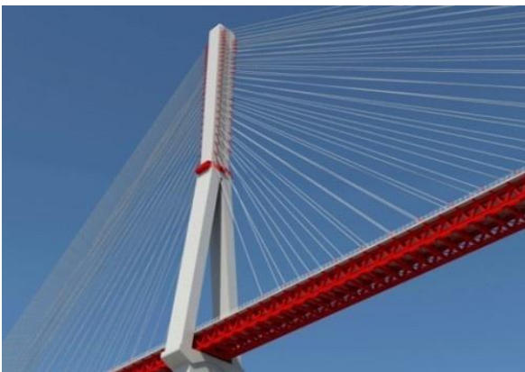
ANJI KHAD BRIDGE
