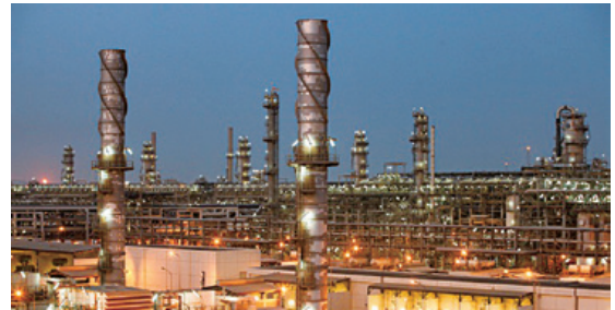
Natural gas liquefaction plant (Qatar)
