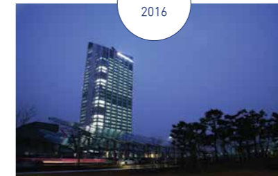
Launched COK11 and was ranked first in the energy/utility sector by CDP
