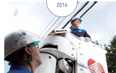
Completed the installation of Saemangeum transmission lines after resolving conflicts
