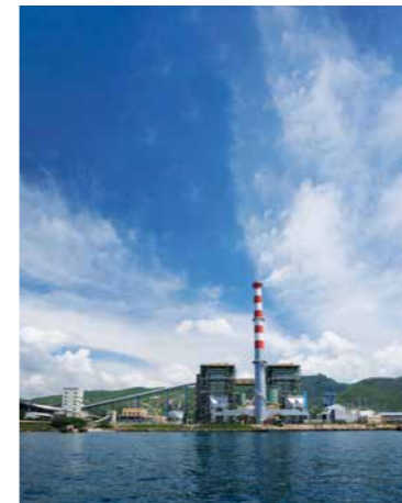
Power plant in Cebu, Philippines
