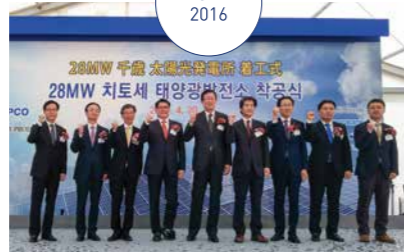
Successfully launched its first overseas solar power plant project
