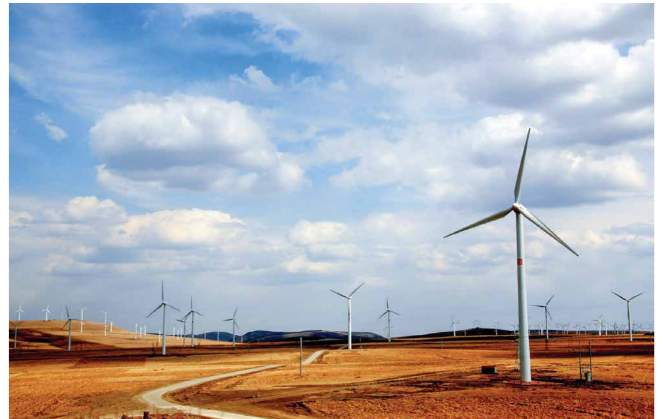
Wind farm in Inner Mongolia, China
