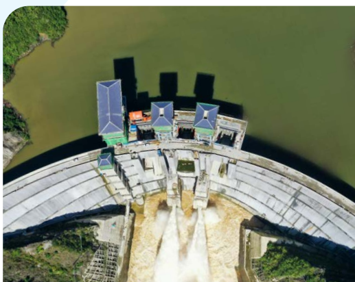
陕西省引汉济渭工程项目 Water Diversion from Hanjiang River to Weihe River in Shaanxi Province
