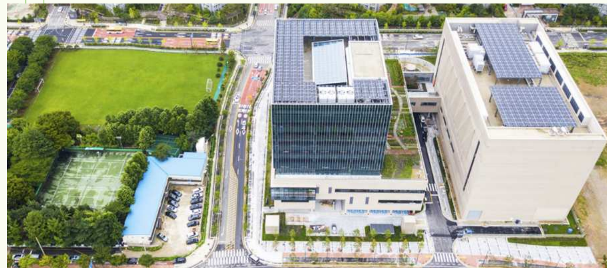
Solar Power System at the KDB Digital Square
