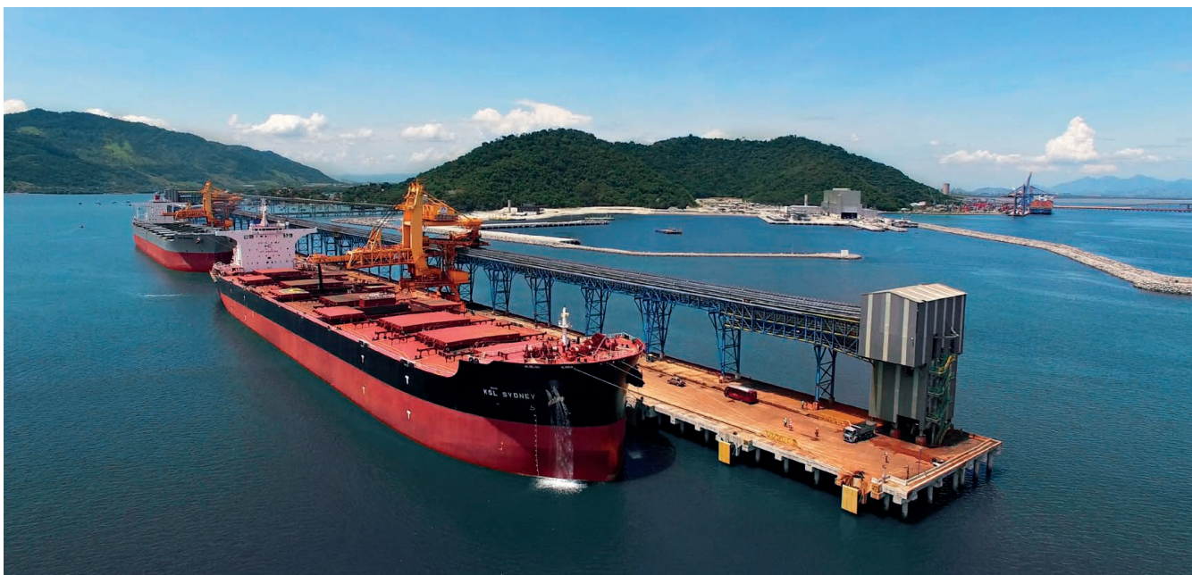
Impala Terminals and Mubadala's Porto Sudeste export facility, Brazil.
