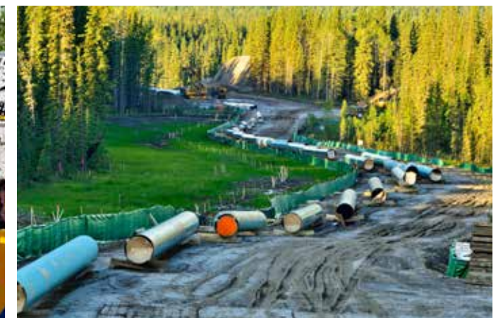
Laying out the Trans Mountain oil pipeline near Hinton Alberta Canada PHOTO: Robert McGouey / Industry / Alamy Stock Photo
