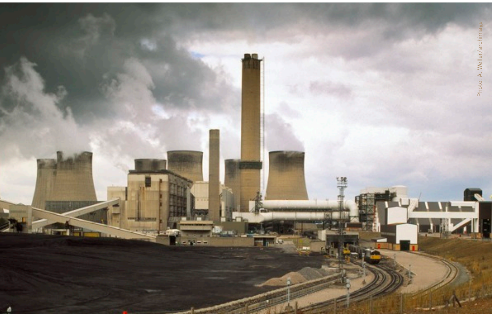
The E.ON plant Ratcliffe-on-Soar is one of the highest CO 2 emitters in Britain. Environmentalists have repeatedly staged blockades to get the plant shut down.
