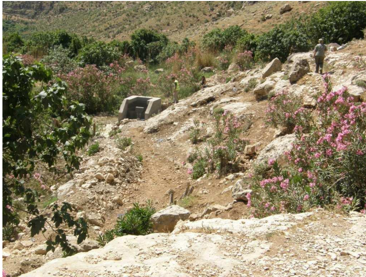
Photo 10: Drinking water intake The site is accessible only by a footpath, the structure is rather small and inconspicuous. May 2008
