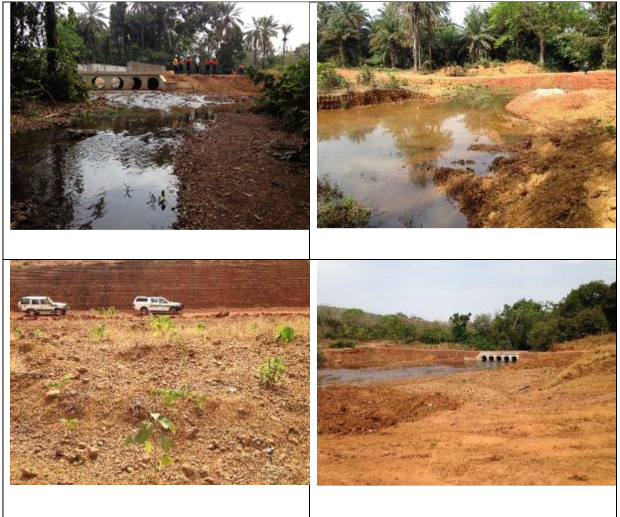
Figure 23: Top left and top right– northernmost river crossing of old COBAD alignment, Bottom left – native tree planting, Bottom right – Southern river crossing of old COBAD alignment.
