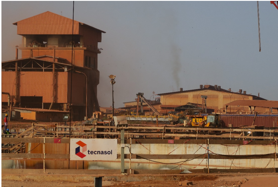
Photo 1. Bauxite crusher pit (foreground) with existing crusher in the background
