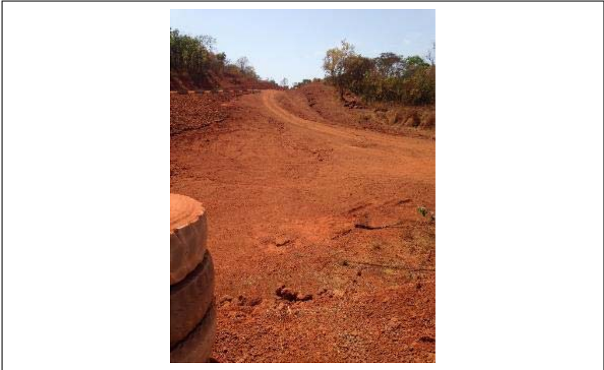
Figure 24: Slope Vulnerable to Erosion Adjacent to Critical Habitat Watercourse
