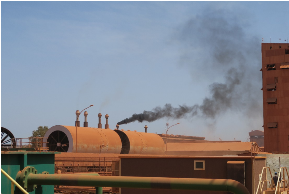
Photo 29. Air emissions during start up of power generating unit following a trip
