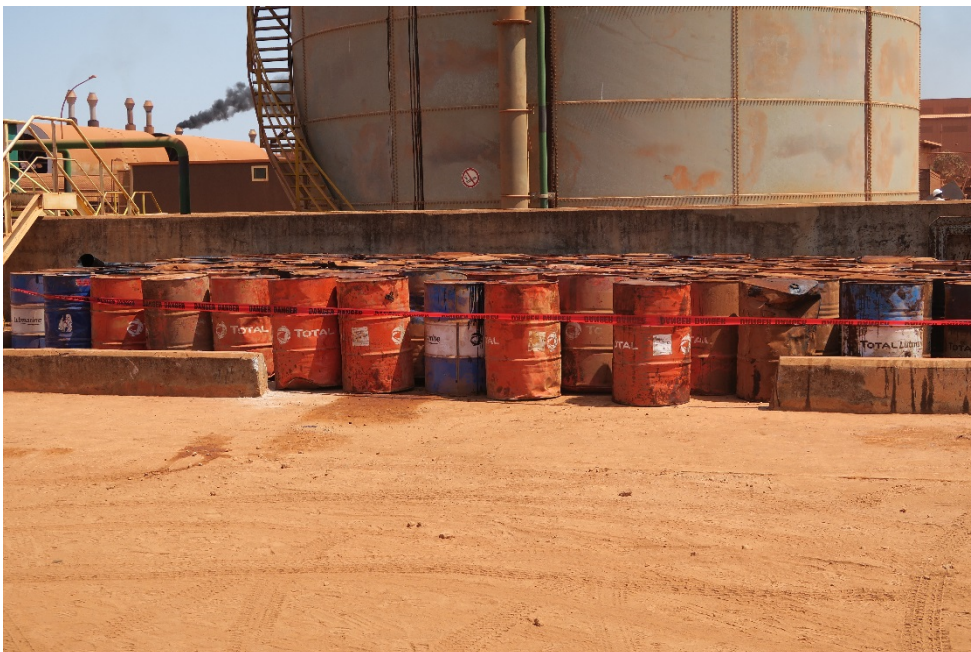
Photo 30. Temporary storage of oil during malfunctioning of oil/water separator. Bund wall removed to allow access.
