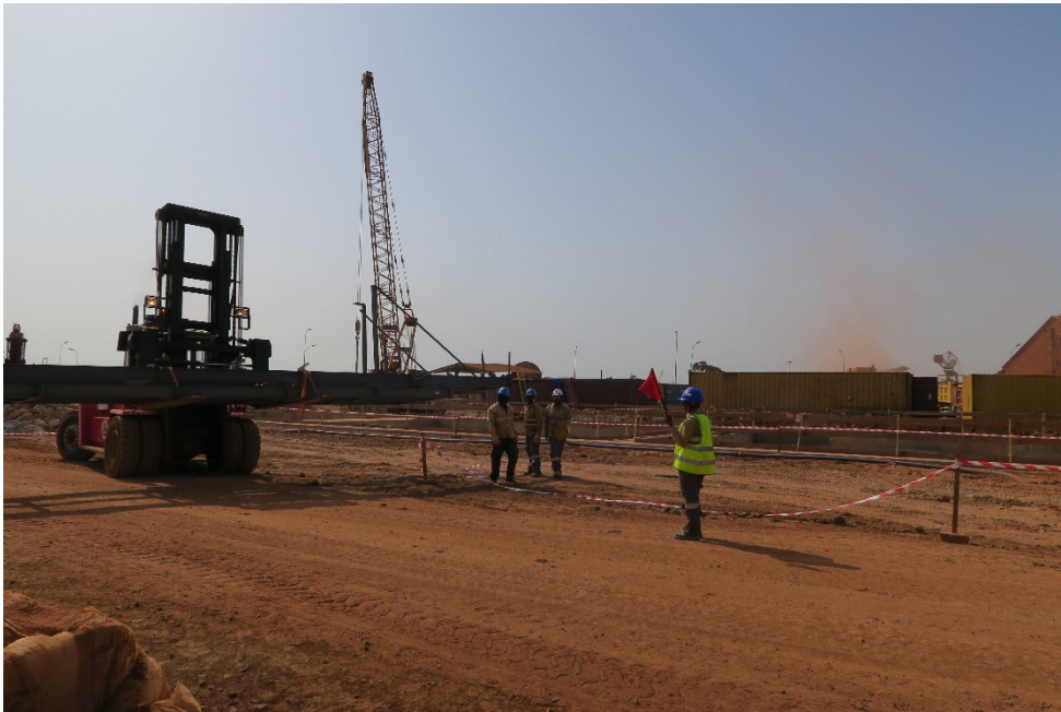
Photo 9. Use of flag man with large plant to mitigate restricted vision
