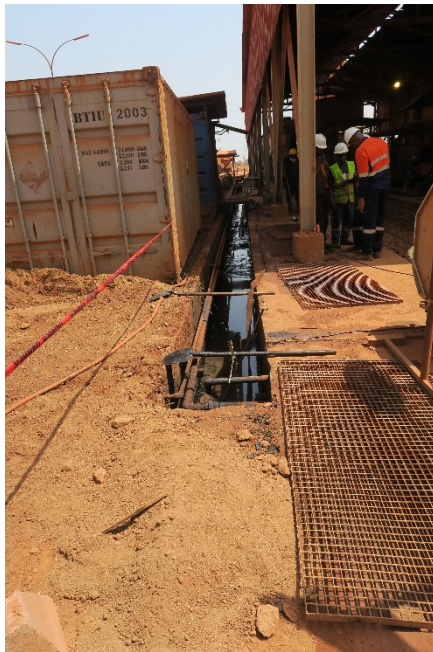
Photo 17. Drainage ditch adjacent to locomotive fuelling area – heavily contaminated with oil
