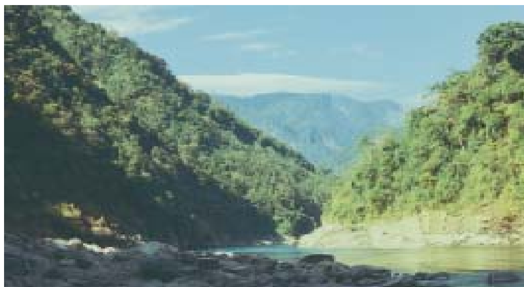
Site of the dam axis (270m high dam), Debang Valley Multipurpose Project, Debang Valley District, Arunachal Pradesh.
