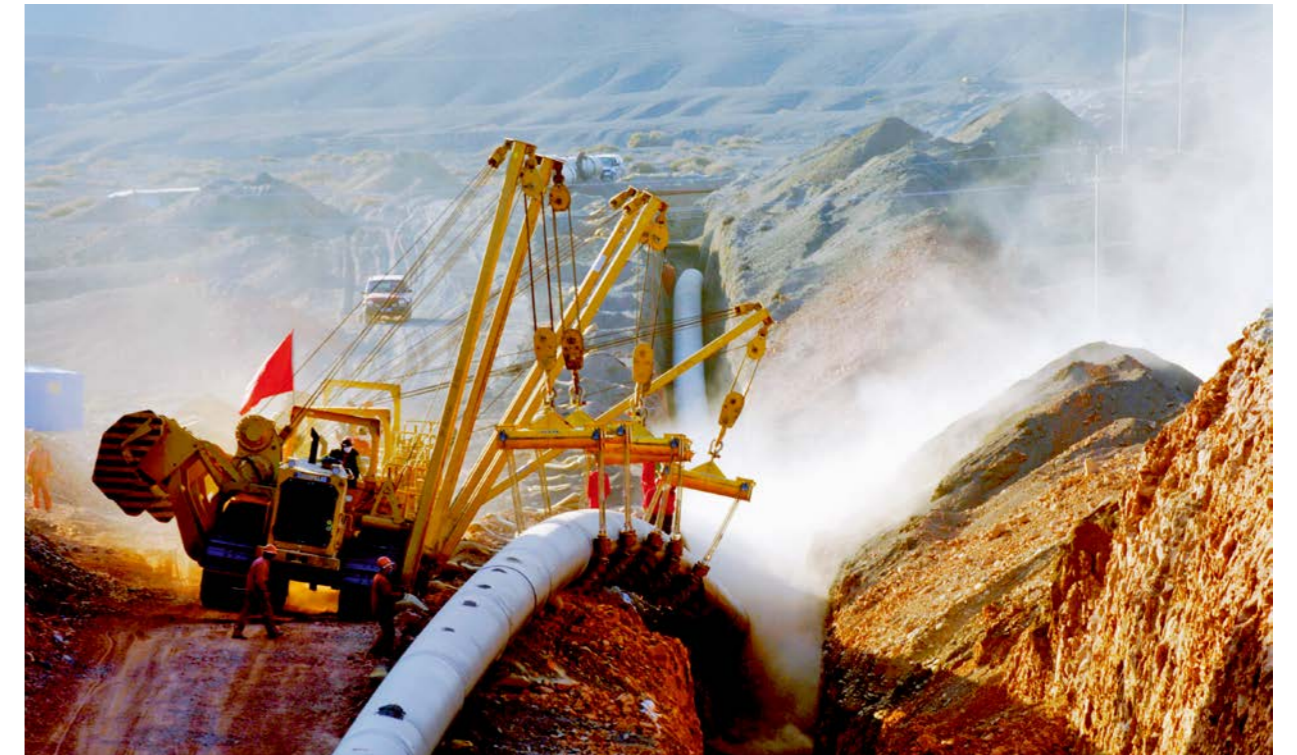
Construction scene of "West-East Natural Gas Pipeline" project
