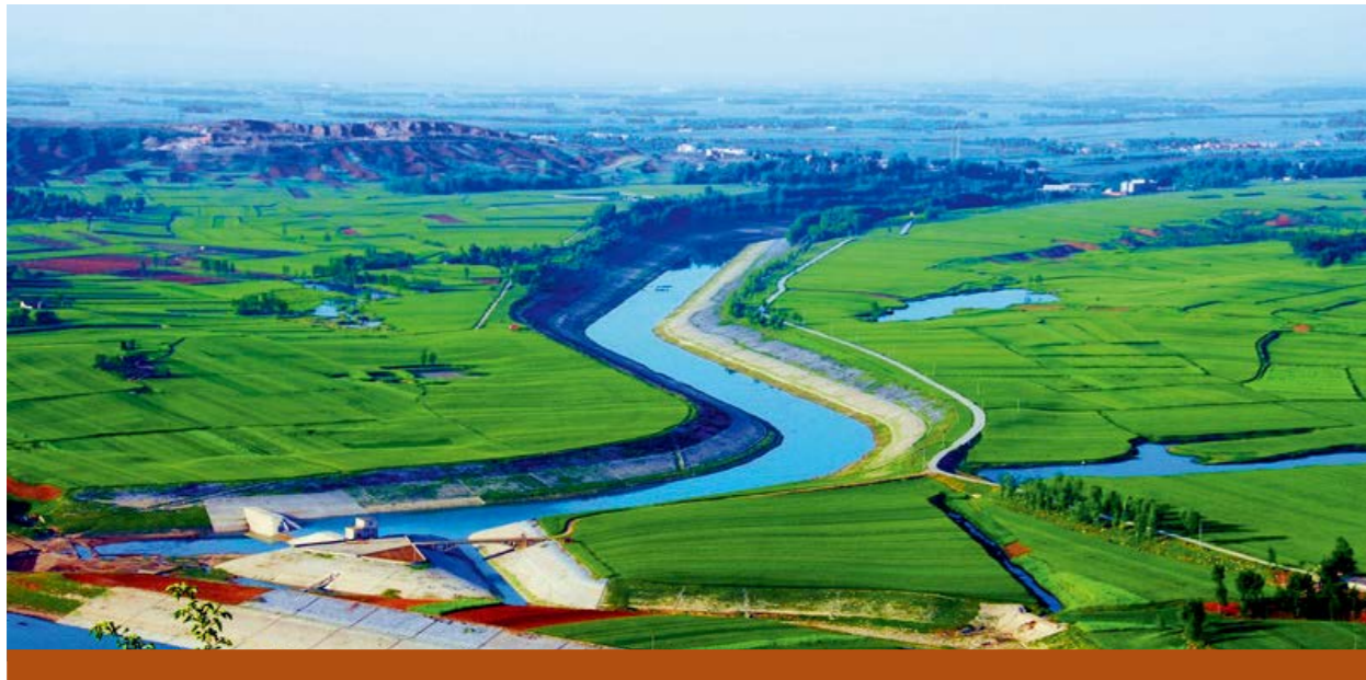
Landscape of the midline channel of the "South-to-North water diversion" project
