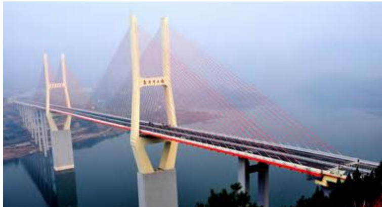
Pengxi River Bridge along the Chongqing-Yibin Expressway.
