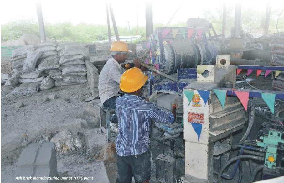
Ash brick manufacturing unit at NTPC plant
