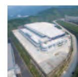
Logistics Republic Zones B3, B3, B6, B5, B7 and Yangmei Zone EEWH Silver Certification
