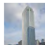
Cathay Landmark EEWH Gold Certification / LEED Gold Certification
