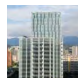
Minsheng Jianguo Building EEWH Diamond Certification / LEED Gold Certification
