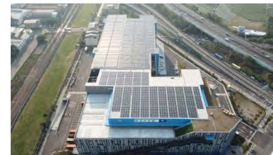
Solar power roof of Logistics Republic Taichung Wuri
