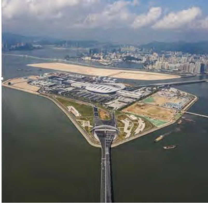
Zhuhai Branch in Guangdong supports the construction of the Hong Kong-Zhuhai-Macao Bridge Artificial Island Port (Photo by Yangjie)
