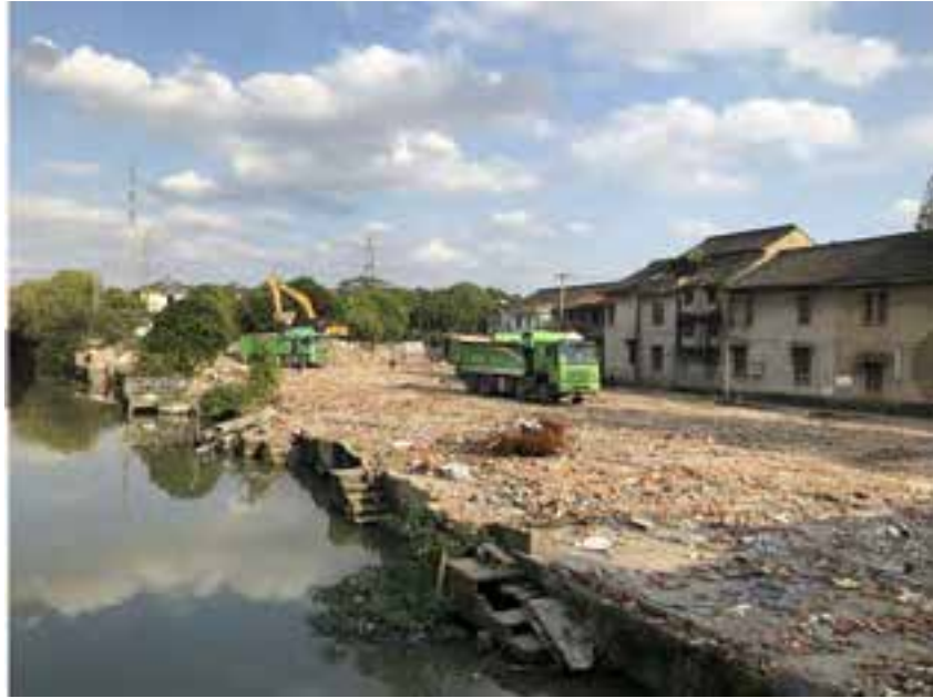
The demolishing old street (Photo by Ni Chenlai)
