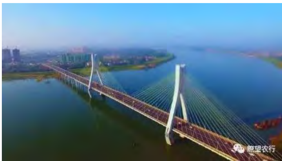
Hunan Branch supports the Spanning Zihe River project during the
