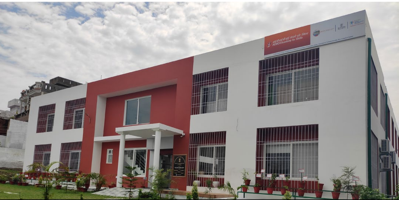
ICICI Academy inaugurated a new centre at Jammu. This is the first Indian Green Building Council certified green building in the UT of Jammu & Kashmir
