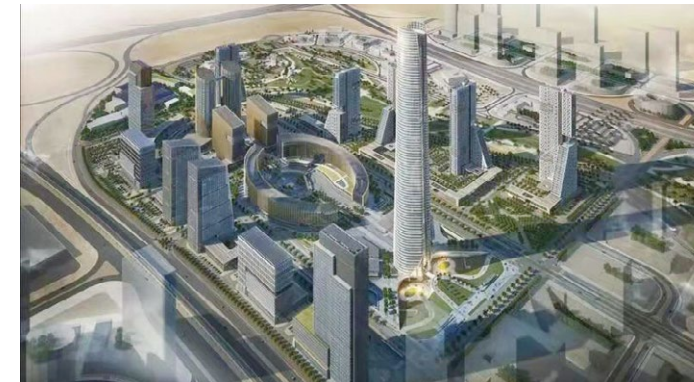
A phase III project of the central business district in Egypt's new administrative capital
