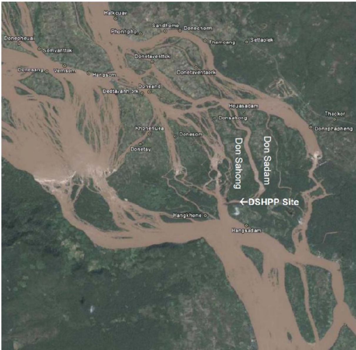
Figure 3-1 DSHPP Site on the Hou Sahong
