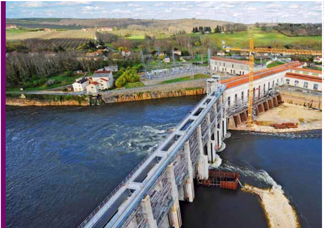
Run-of-river dam at Tuillières, on the Dordogne. Part of the SuperHydro (hydro safety and performance) program involving 450 projects to renovate and modernize the hydro fleet in France.
