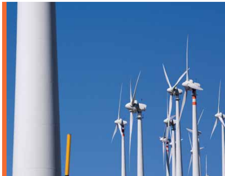
Wind turbines at Castiglione Messer, in Italy. In 2007, Edison brought 10 MW of wind power into service and an additional 84 are being built.
