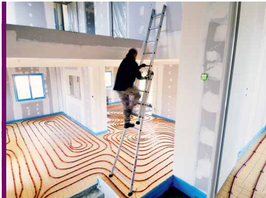
Installation of floor heating system linked to a heat pump. EDF is now delivering comprehensive solutions including insulation and heating systems based on renewable energies.
