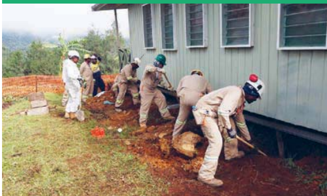
Volunteers repair foundations at Para Primary School
