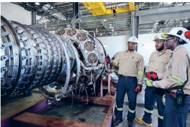
Mechanical Technician, Junias Warpin, Machinery Engineer, Jimmy Simatab and Operations Technician Level 1, Julian Romel, inspect a gas turbine at the LNG Plant
