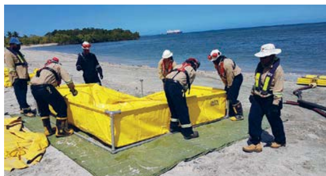
Setting-up temporary waste storage for recovered oil and wastewater during a shoreline response drill
