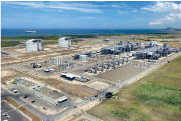
Aerial view of the LNG Plant
