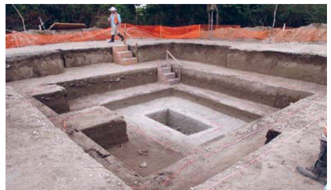
An excavation site at the LNG Plant uncovered during the construction phase of PNG LNG
