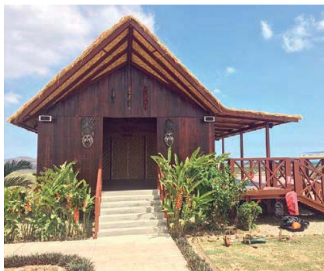
| The renovated LNG Plant observation deck
