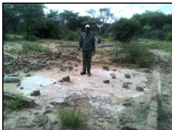
Cement foundations at ruin 1.
