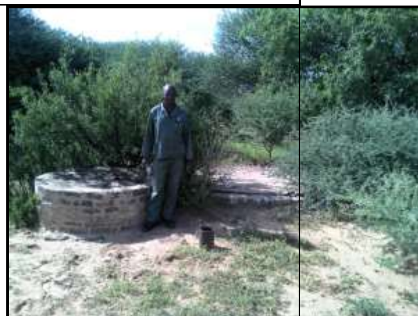
Cement and brick foundations of waterhole at ruin 1.
