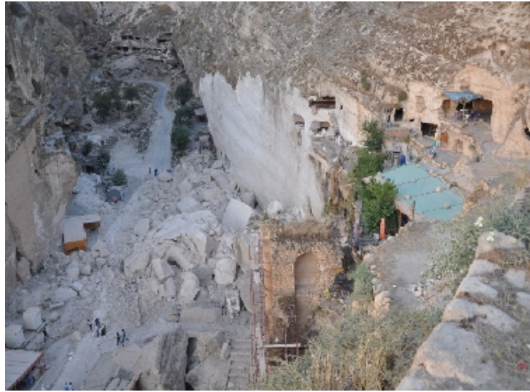
Situation one day after the rock fall
