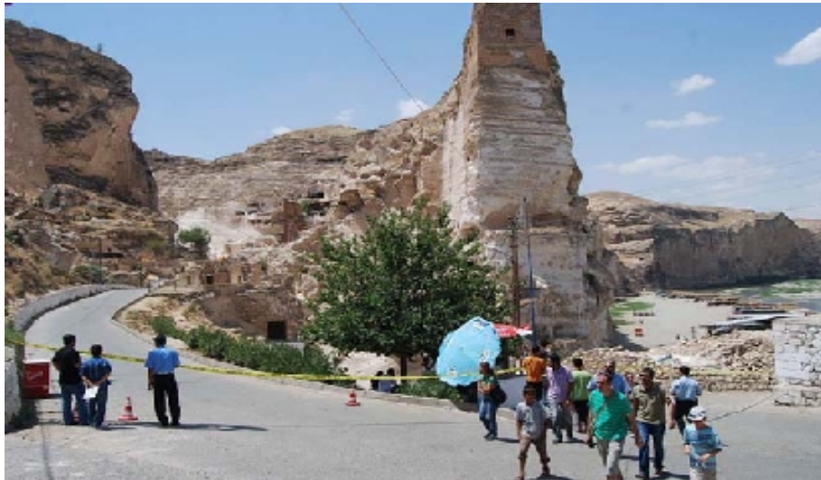
After the rockfall the acces to the castle and the surrounding area has been forbidden
