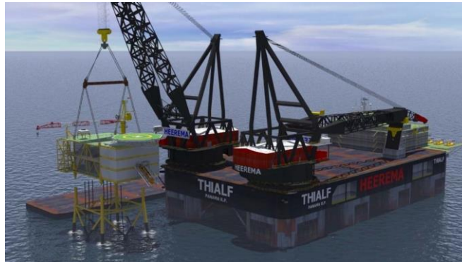
Figure 2-11 Typical topsides lift by a HLV (example HLV).
