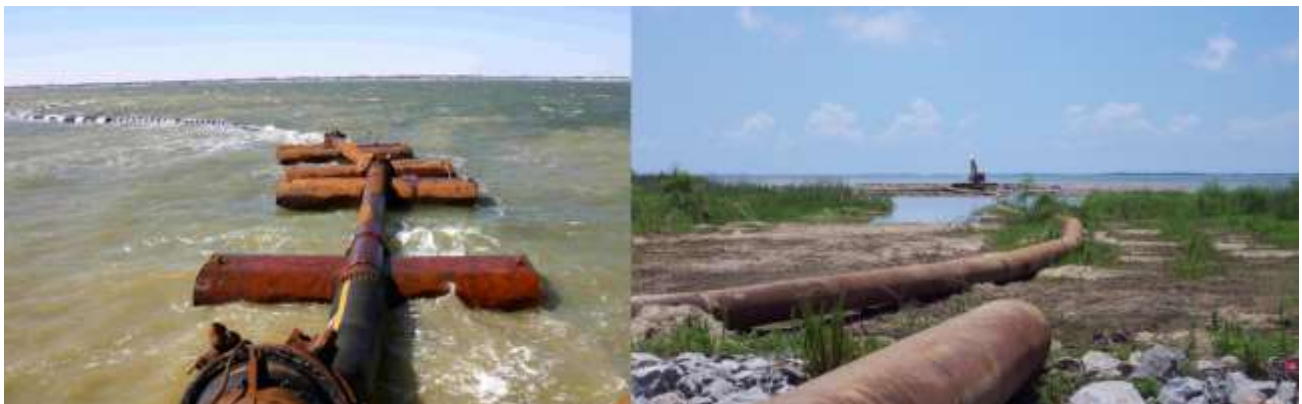
Figure 5: Dredge line on water (floating) and on land (Right)
