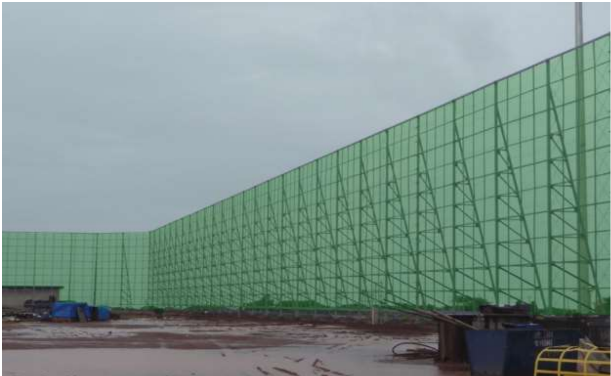
Figure 8: Windshield around the port as a second line of defense against dust emission
