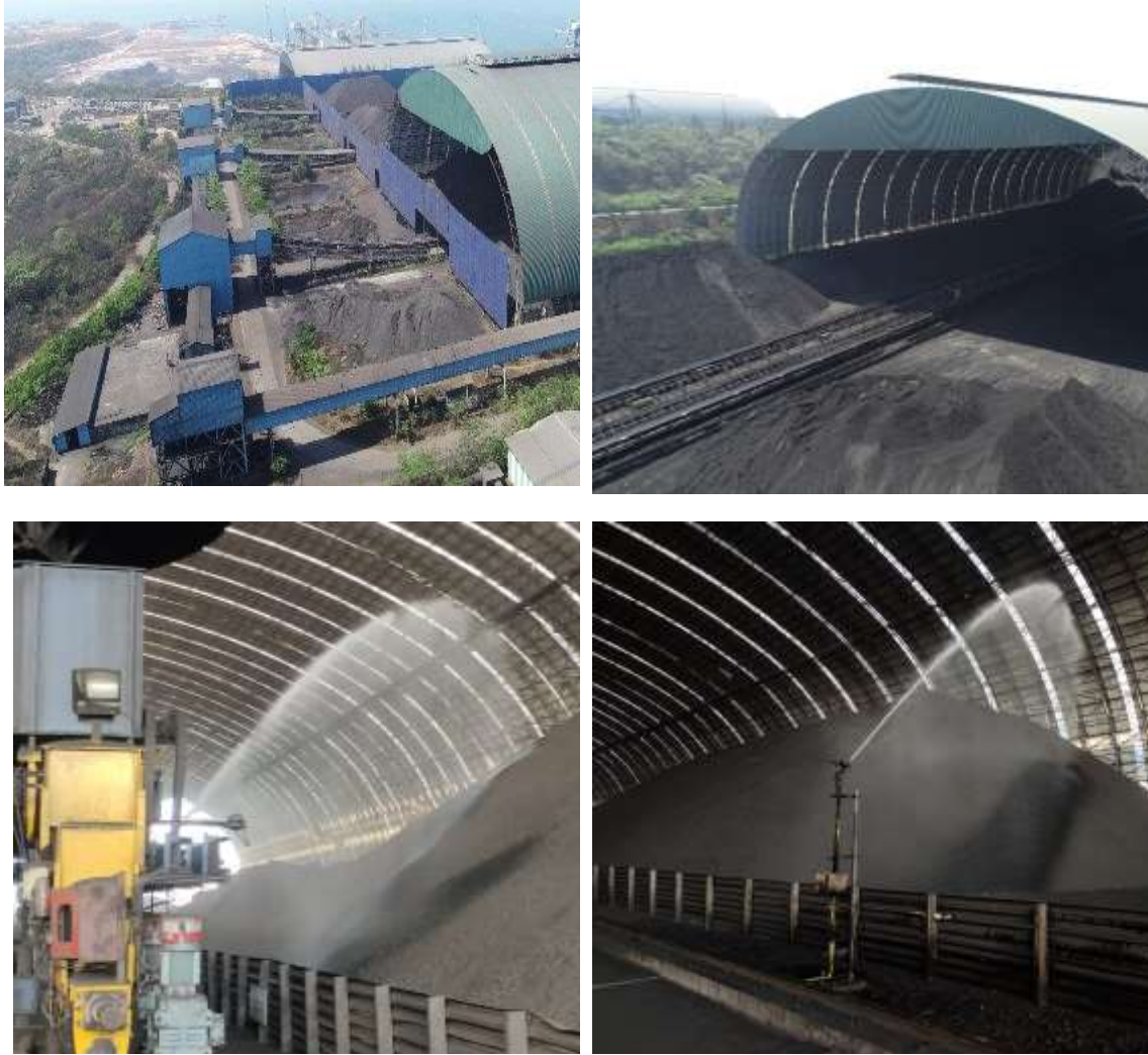
Figure 9: Longitudinal Cover shed with DSS
