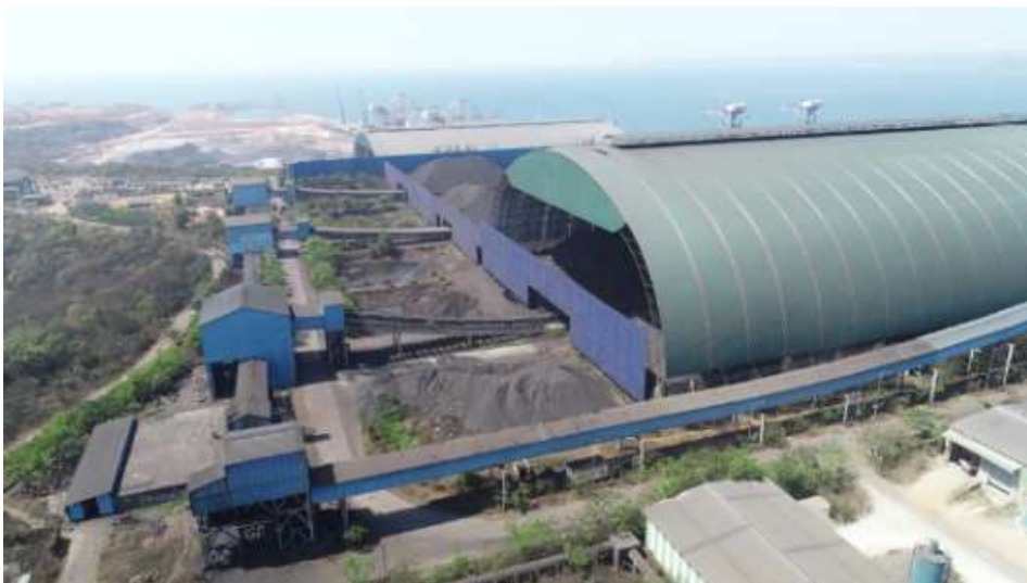
Figure 5: Covered conveyors conveying the material in to the covered storage
