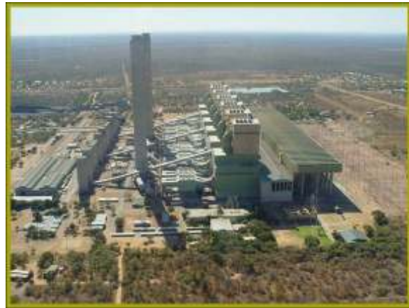
Photo 2.2 Direct dry-cooled power station
