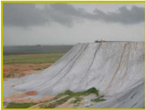
Photo 4 Above-ground ash dump
