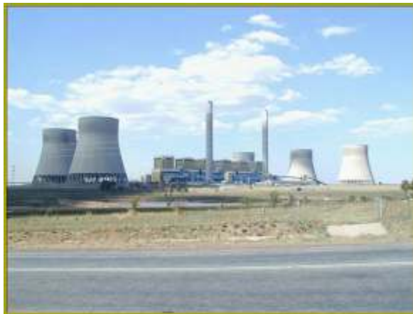
Photo 2.1 Indirect dry cooled power station
