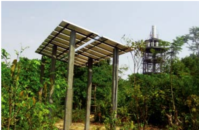
Solar Panels in Kampot Province Used to Run a Solar Pump, which Fills the Water Tower in the Background. Photo courtesy of Clean Energy Group.
