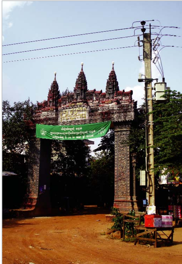
A Transmission Line in Cambodia. Photo courtesy of International Rivers.
