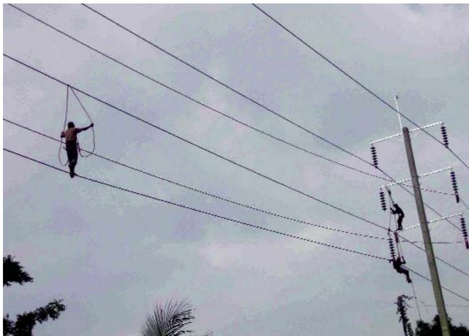
Constructing the Mekong Power Grid Transmission Line
