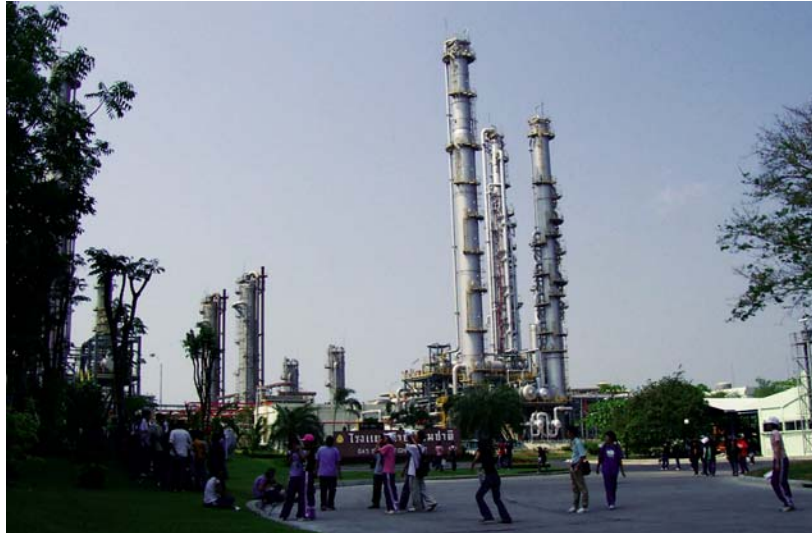
A Natural Gas Separation Plant in Rayong, Thailand.
