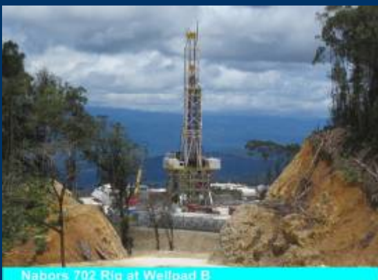
Nabors 702 Rig at Wellpad B
