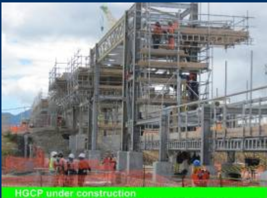
HGCP under construction
