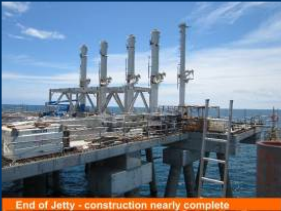
End of Jetty - construction nearly complete
