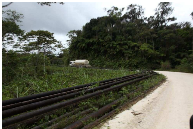
Pipe lines of existing oil facility running around Lake Kutubu Credit: Damian Baker
