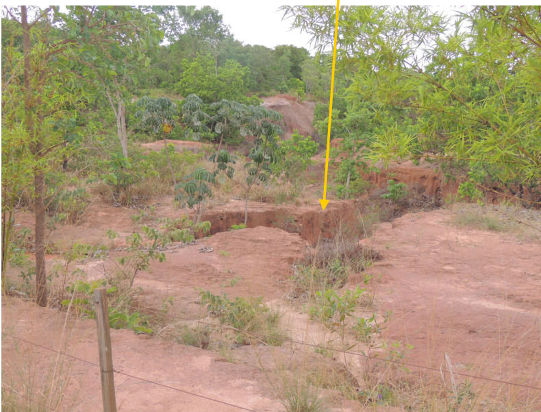
Photo of the area on MS 444 road where there are big cracks in the ground. Coordinates -20°10'52, -51°47'22.
