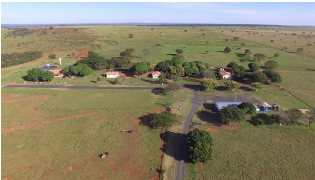
Example of a cattle ranching farm in Mato Grosso do Sul, with main house, employees' houses and other buildings.
