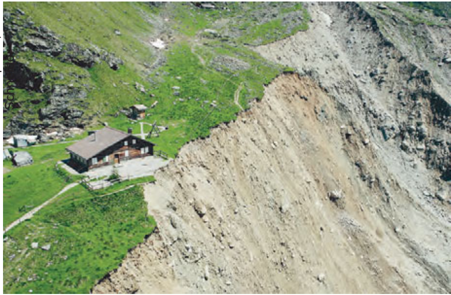
Landslide in Switzerland as a result of excessive rainfall
