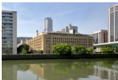
Osaka Head Office with renovations completed
