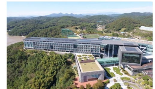
Solar power generation facility at the KB Insurance training institute
