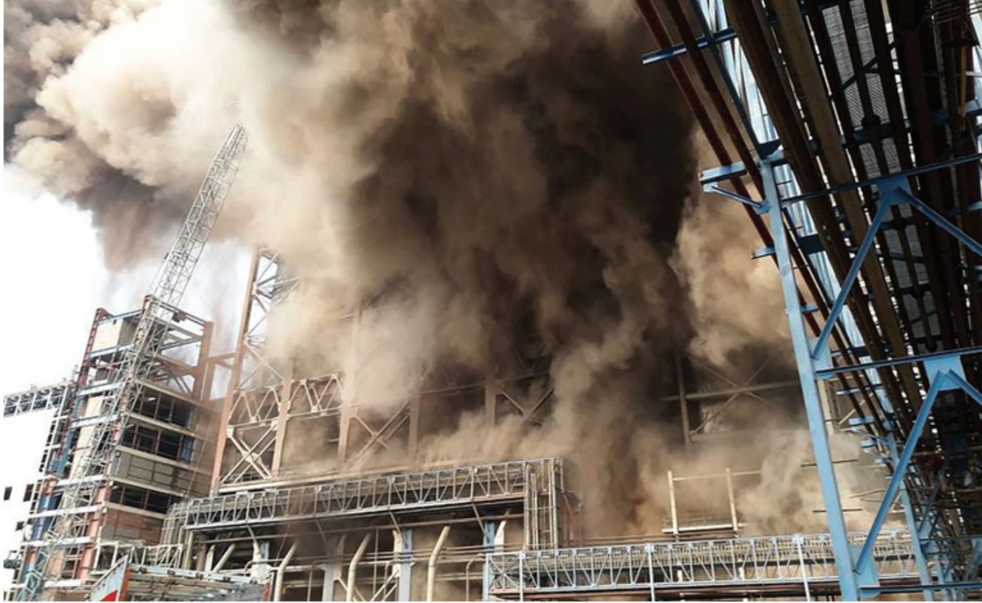
▲ Visual after the boiler blast at Unchahar Power Plant, Uttar Pradesh (Source: Bloomberg Quint)
