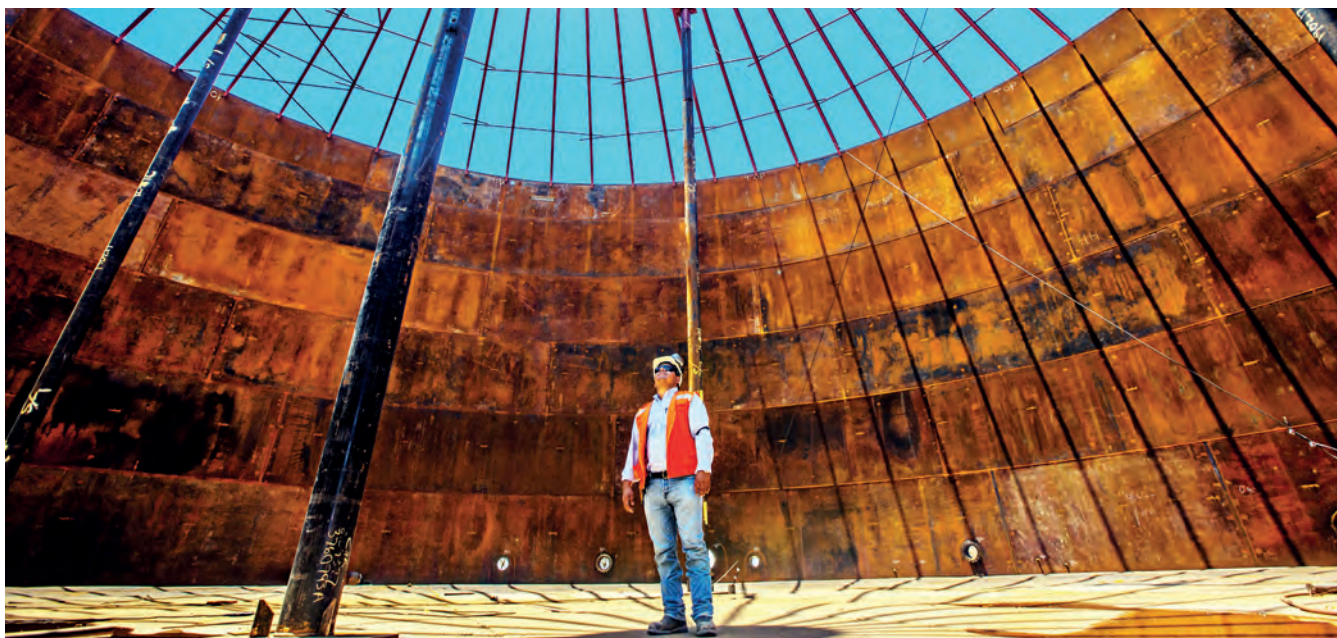
Fuel storage construction, Impala Terminals' Barrancabermeja facility, Colombia.
