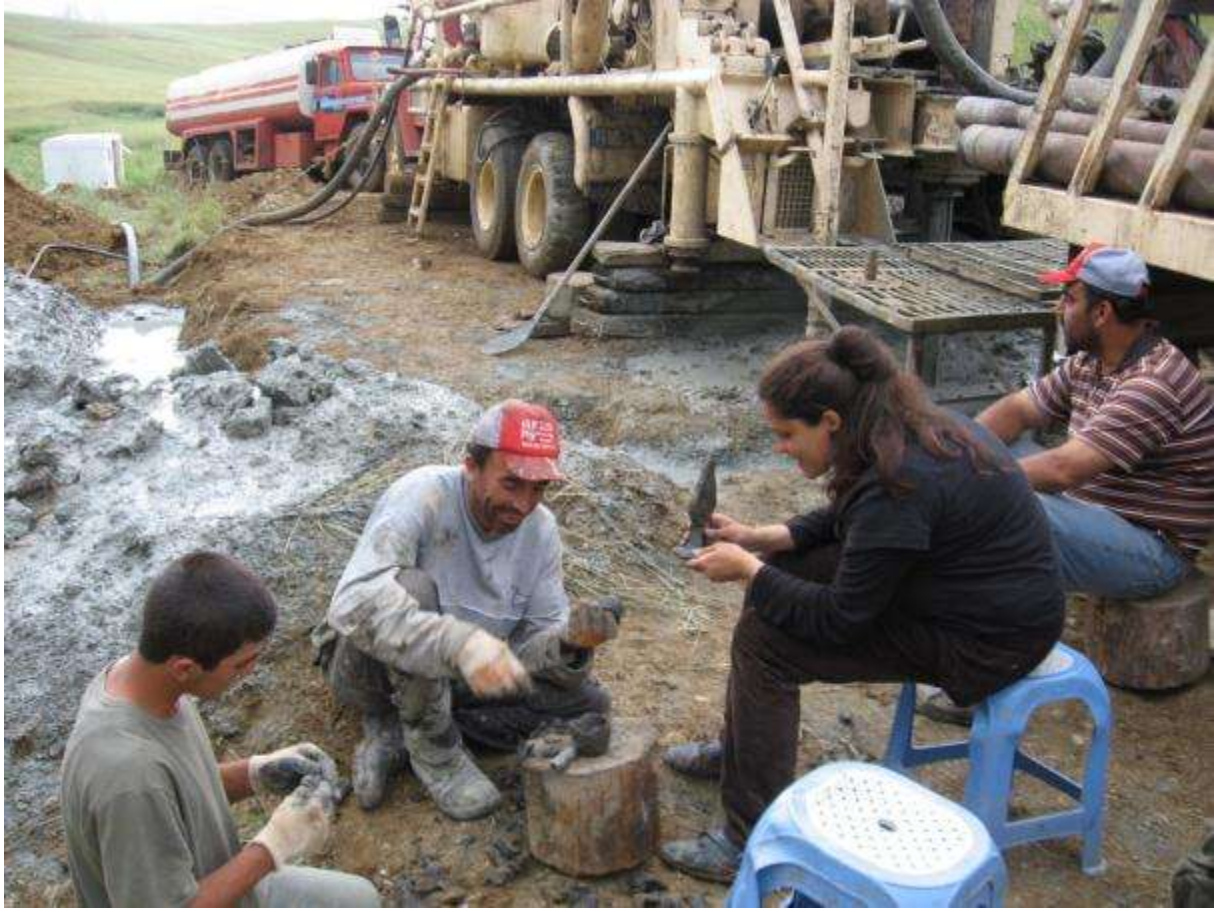
Photo 7: Enerjisa Project Engineer together with workers during performing boreholes
