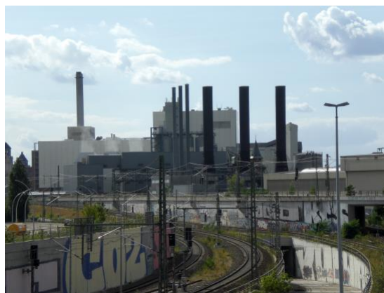
Moabit power and heat plant, Photo: Wikimedia
