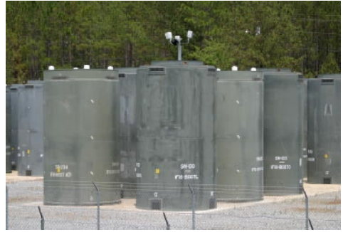
Dry storage at Plant Hatch
